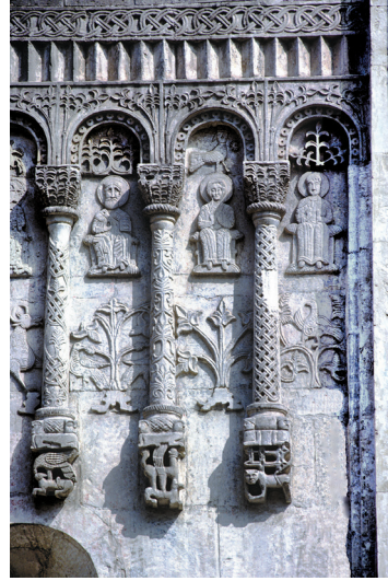
19A. Cathedral of St. Demetrius, west façade, north bay, right side. Center: seated figure of Theotokos. Brumfield. 26/4/1980
